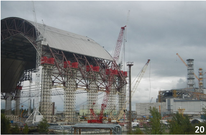
September 2013: Third lifting operation for the first half of the arch.
