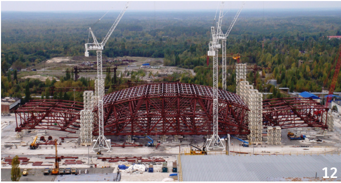
October 2012: Assembly continues.
