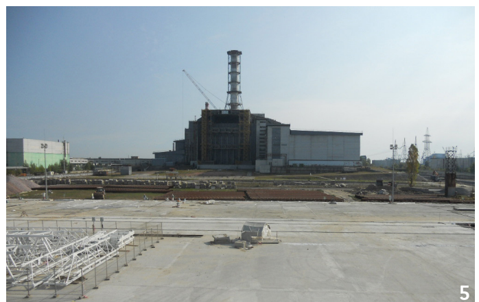
5 September 2011: Start on assembly preparatory work.
