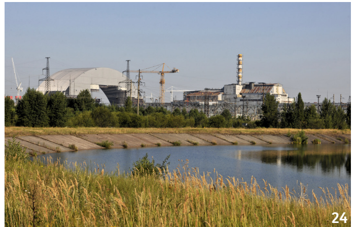
August 2014: Second lifting operation for the second half of the arch. ©Francis Vigouroux
