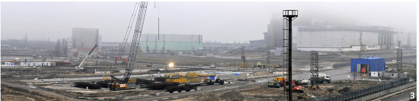
3 August 2010: Start on the foundations for the lifting towers. - ©Francis Vigouroux
