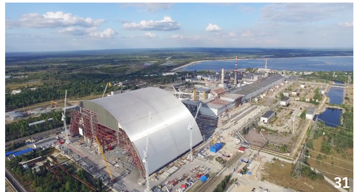
October 2015: Interconnection of the two halves of the arch.
