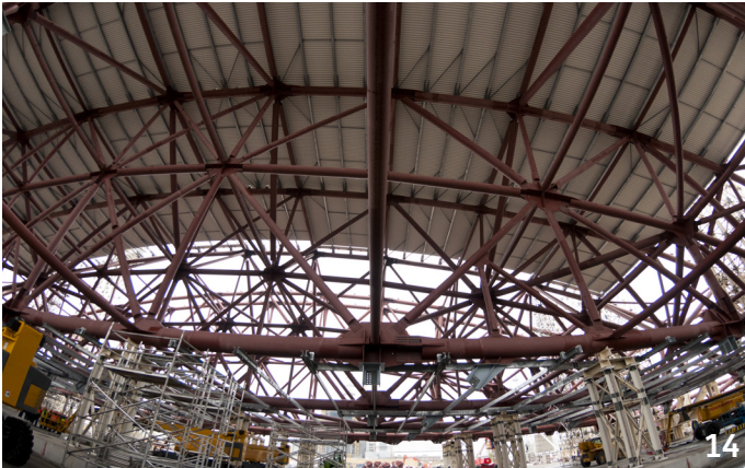
October 2012: The cladding starts with the installation of the purlins and complex wall system. - @Guillaume Daveau
