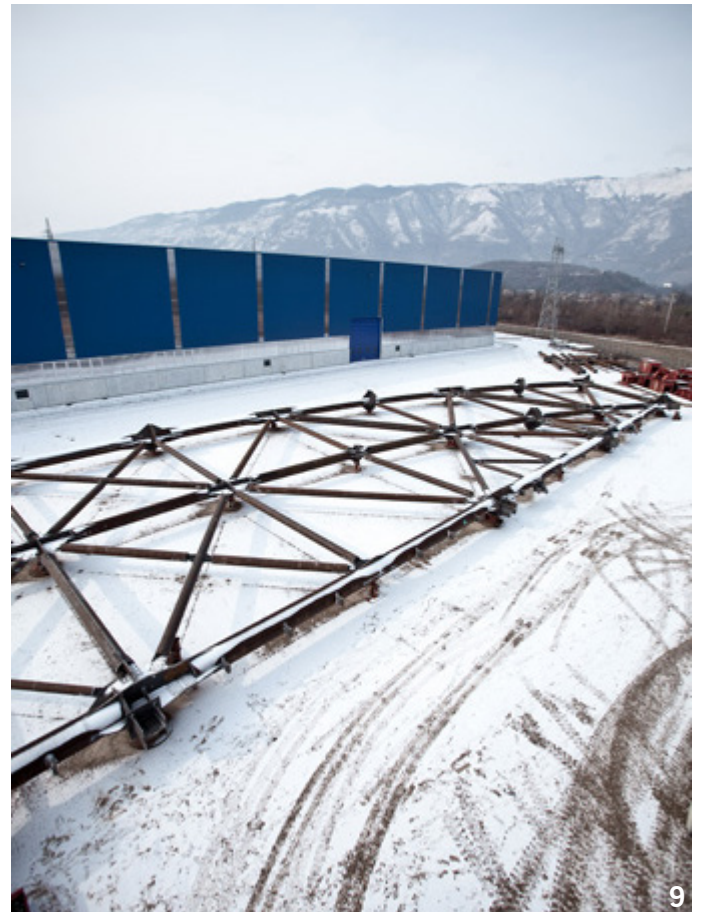
9 February 2012: Assembly test at the Cimolai plant in Italy.
