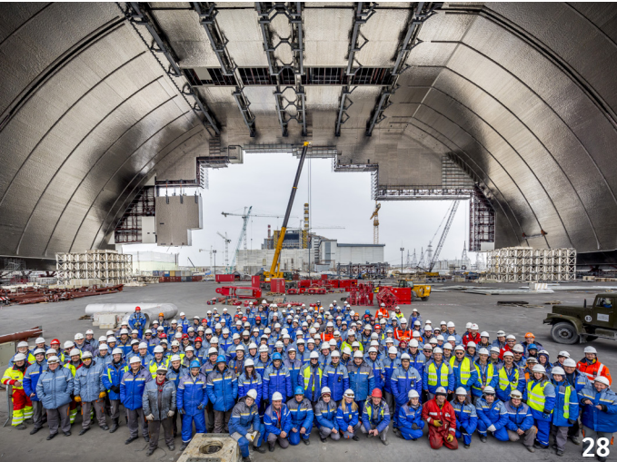
May 2015: Five million accident-free hours worked.
