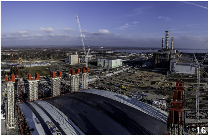
November 2012: First arch lifting operation. - @Jean-Yves Govin Sorel
