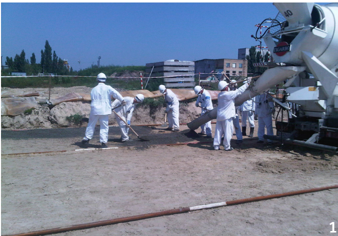
1 Early 2010: Clearing and cleaning the assembly area.
