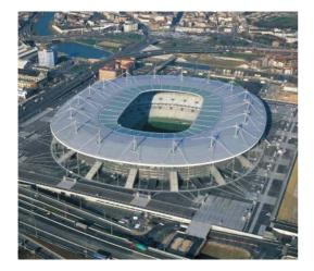
Design, construction, operation and maintenance of a stadium with 80,000 covered seats and a total of  $36,000 \text{ m}^2 \times \text{ of net usable surface}$ . Built on a 14-hectare site, the Stade de France features an elliptical disk-shaped roof suspended 42 metres above the pitch. The playing surface is sunk below natural ground level, reducing the external height of the imposing stadium.
