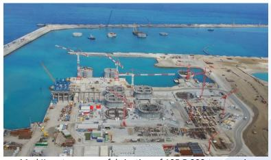
Tanger Med II port: mass prefabrication of 105 5,000-tonne caissons
