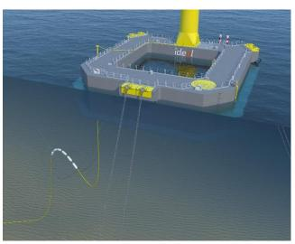
The floating foundation used for FLOATGEN is derived from a concept developed by the French start-up, Ideol. The company has patented a ring-shaped foundation system open in its centre (known as the Damping Pool®), which provides optimal stability at low cost.
